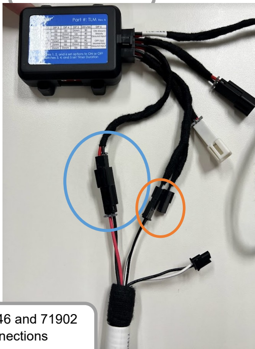
74546 fed through firewall, connected to TLM
