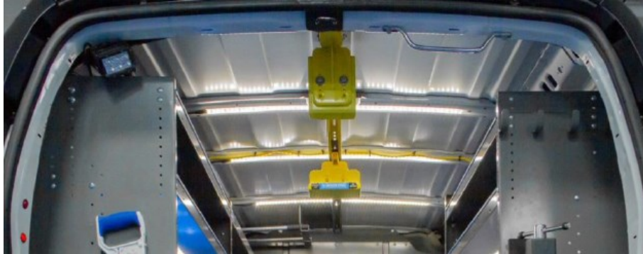
LED Light Strips Installed on Roof Bows
