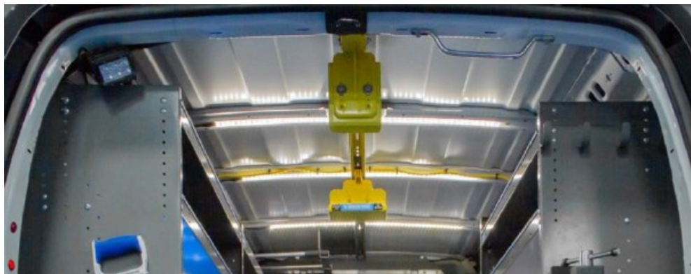
LED Light Strips Installed on Roof Bows
