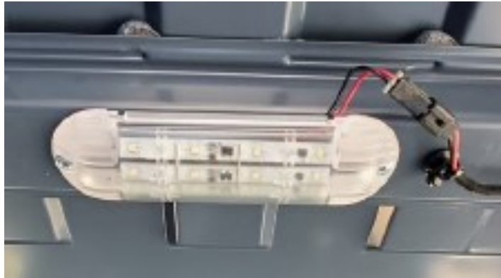
LED Dome Light Installed on Roof Bow
