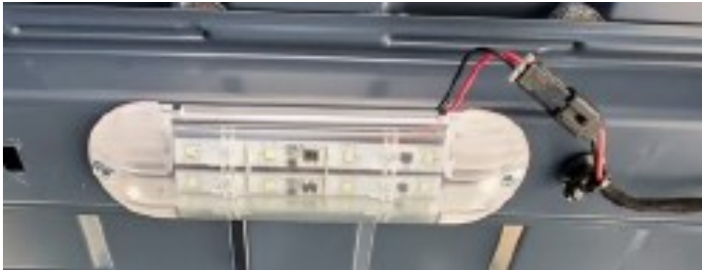
LED Dome Light Installed on Roof Bow
