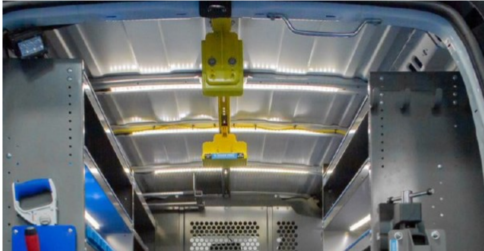
LED Light Strips Installed
