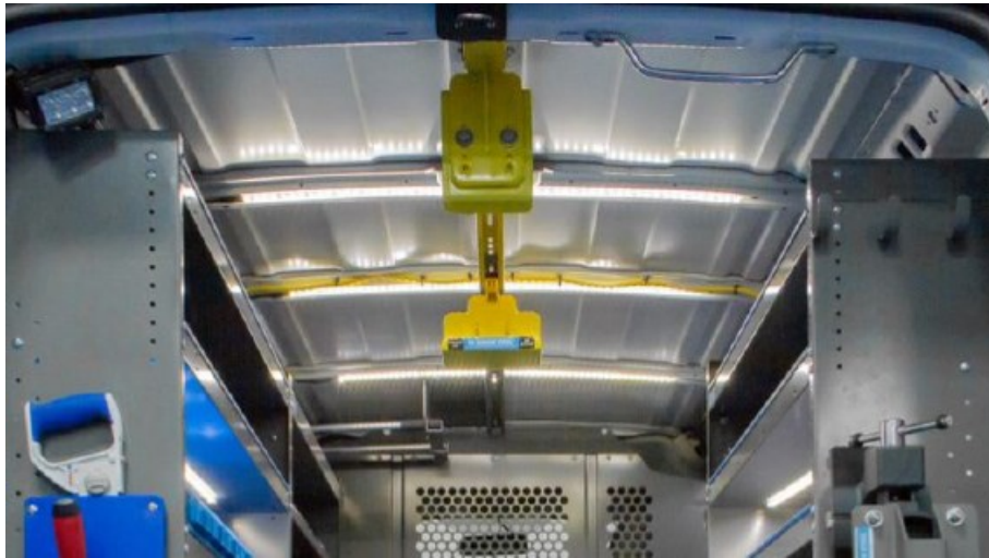
LED Light Strips Installed
