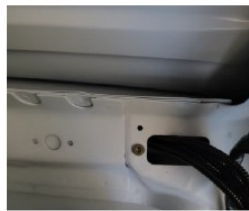
Excess rear switch harness to be tucked in cavity in pillar above rear switch
