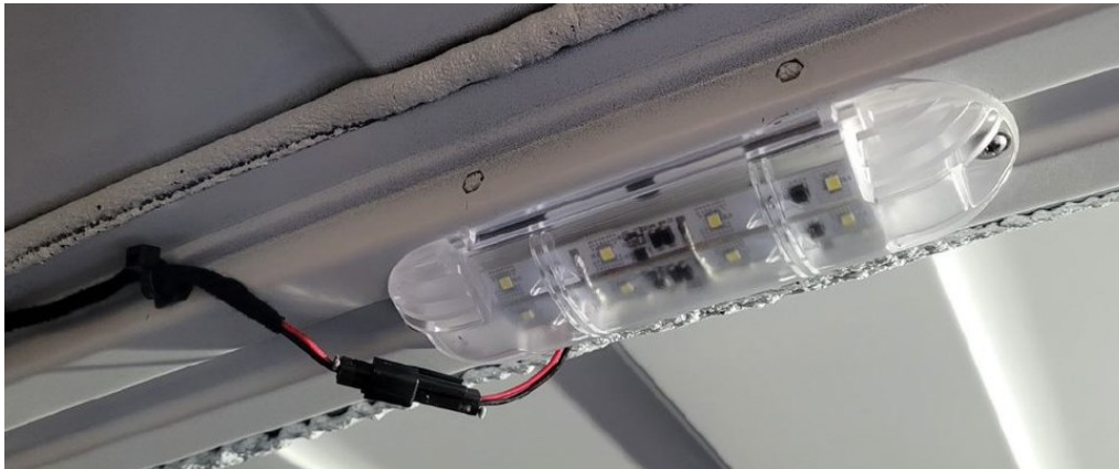
Plug and play LED Module Light Installed
