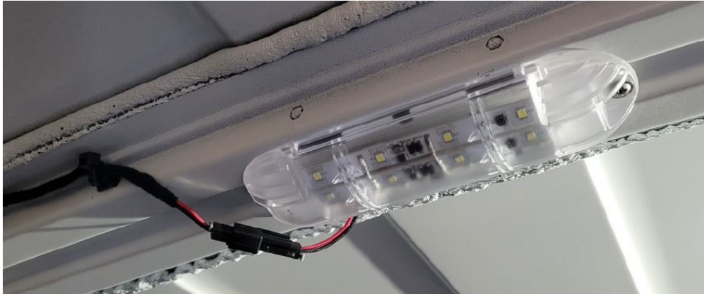
Plug and play LED Module Light Installed
