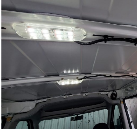
LED Dome Lights Installed on Roof Bows
