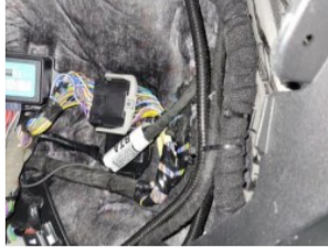
Harness ran up the passenger kick panel and into the A pillar
