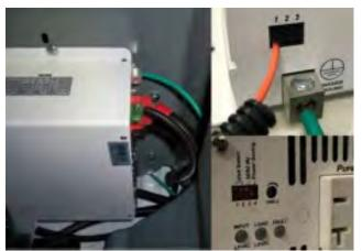
Attach the cables to the inverter
