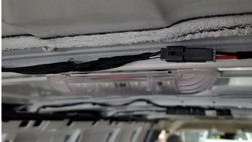
OEM Replacement Light Installed in Cargo of Van
