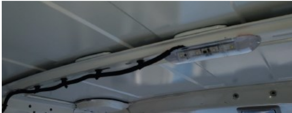
LED Dome Light Installed on Roof Bow
